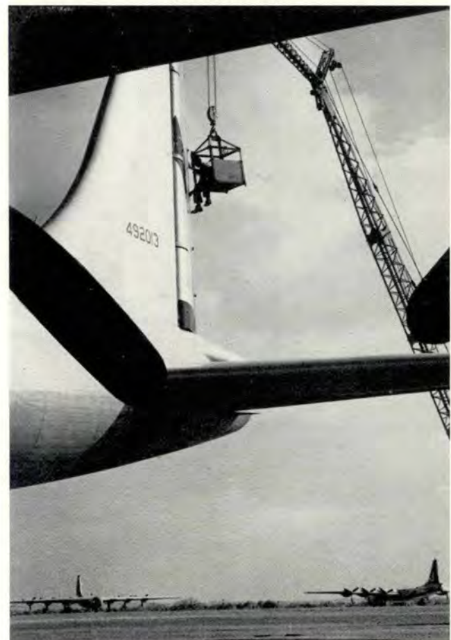
Below: It takes a mobile scaffolding rig to work on a rudder four stories high.
