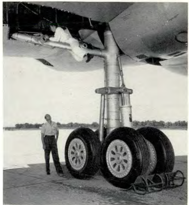
Above: The huge "skate" gear of the B-36 spreads the plane's weight over a larger area.
